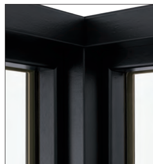
INTERIOR CLOSE UP
