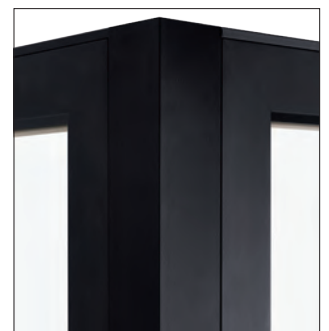
EXTERIOR CLOSE UP
